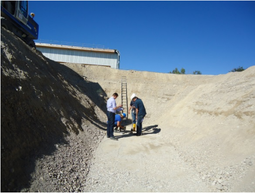
Compaction survey of aviation jet fuel tank excavation (left), placing of aviation jet fuel tank (right)
