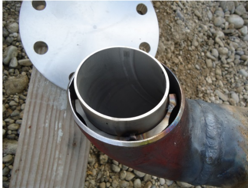
Backfilling compaction (left), safety piping system (right)
