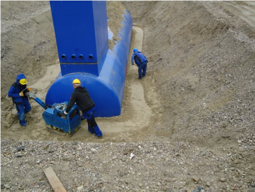
Compaction survey of aviation jet fuel tank excavation (left), placing of aviation jet fuel tank (right)
