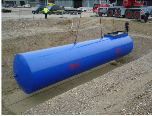
Compaction survey of aviation jet fuel tank excavation (left), placing of aviation jet fuel tank (right)
